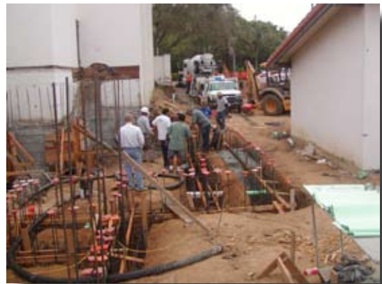
Foundation Work for the Edmundson Terrace photo by Ken Ralph
